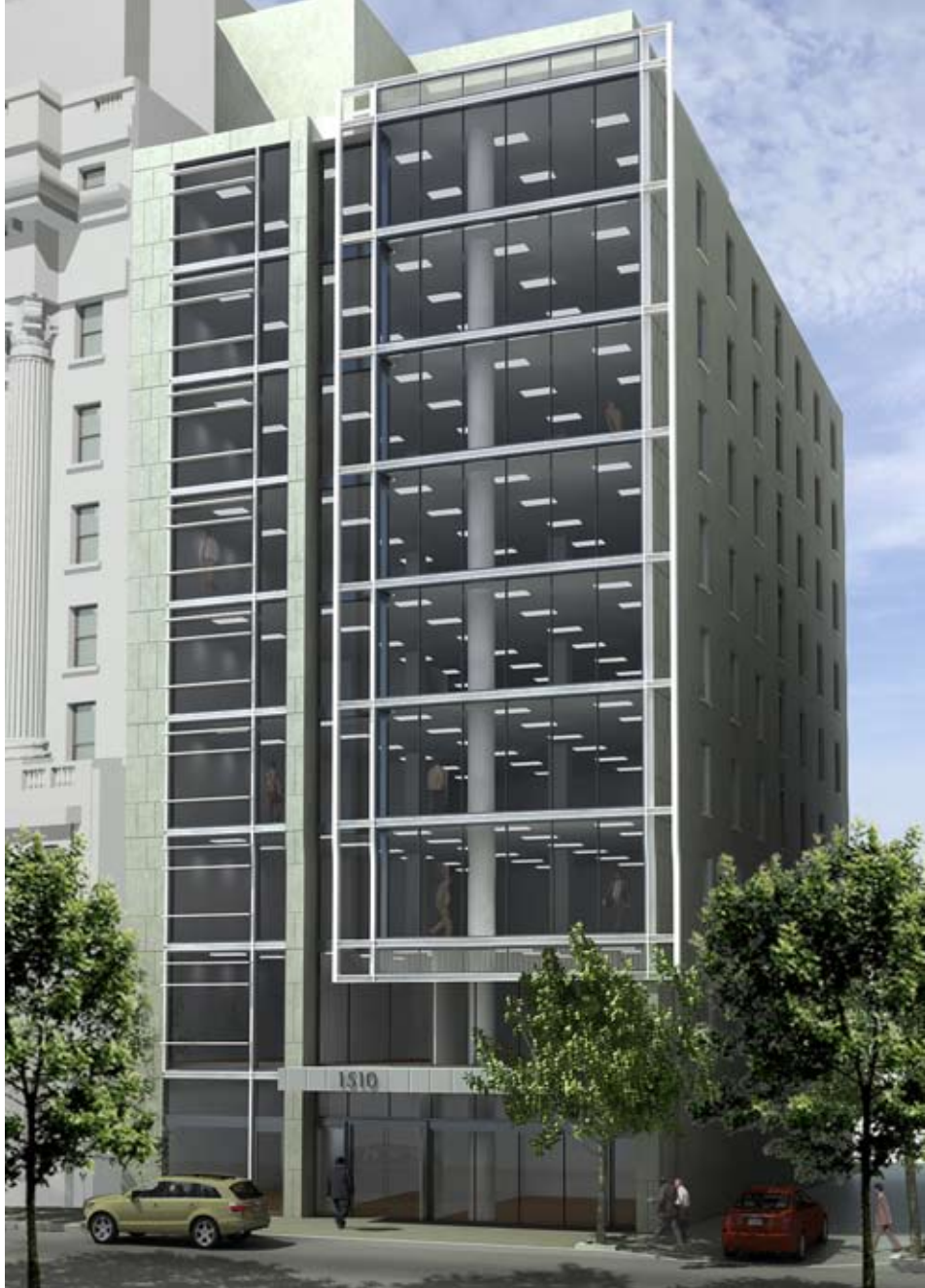
1510 H Street, Washington, DC. This project included demolition of all interior finishes, replacement of existing utilities, building a façade and a multi-level basement parking garage.
